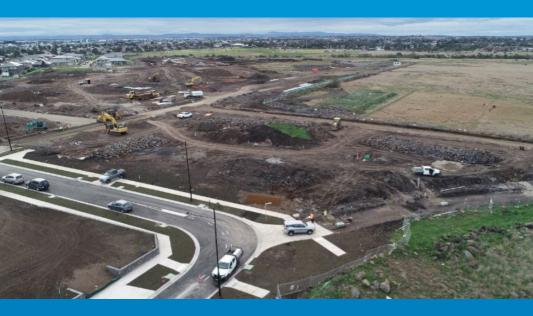
With civil construction progressing well, we anticipate land in Stages 20, 21 and 22 will title in the first half of 2022. Stage 20 concrete kerb and channel works are advancing. Sewer and water reticulation works are underway in Stage 21, and drainage works have commenced in Stage 22.
